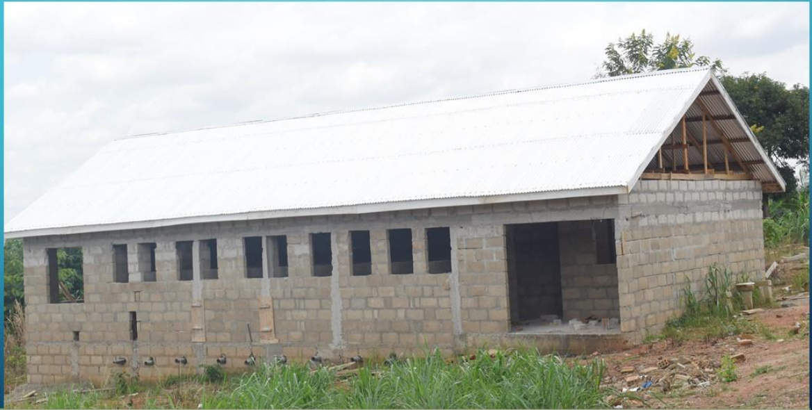
CONSTRUCTION OF 20 SEATER TOILET & BATHROOM AT ADUMAN SHS, ADUMAN
