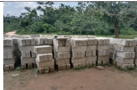
LAYED BLOCKS FOR THE CONSTRUCTION OF THE CLASSROOM BLOCK AT ADADEKROM
